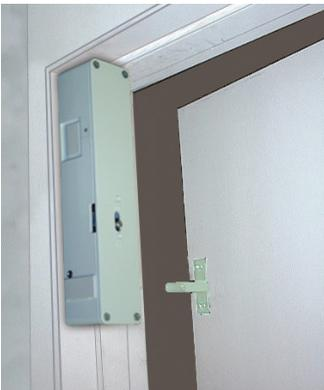
Keeps the hoistway door locked when the car is not there.
