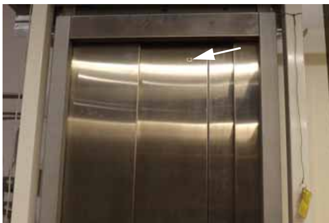
Figure 4: Auto Slim Landing Doors Emergency Opening
